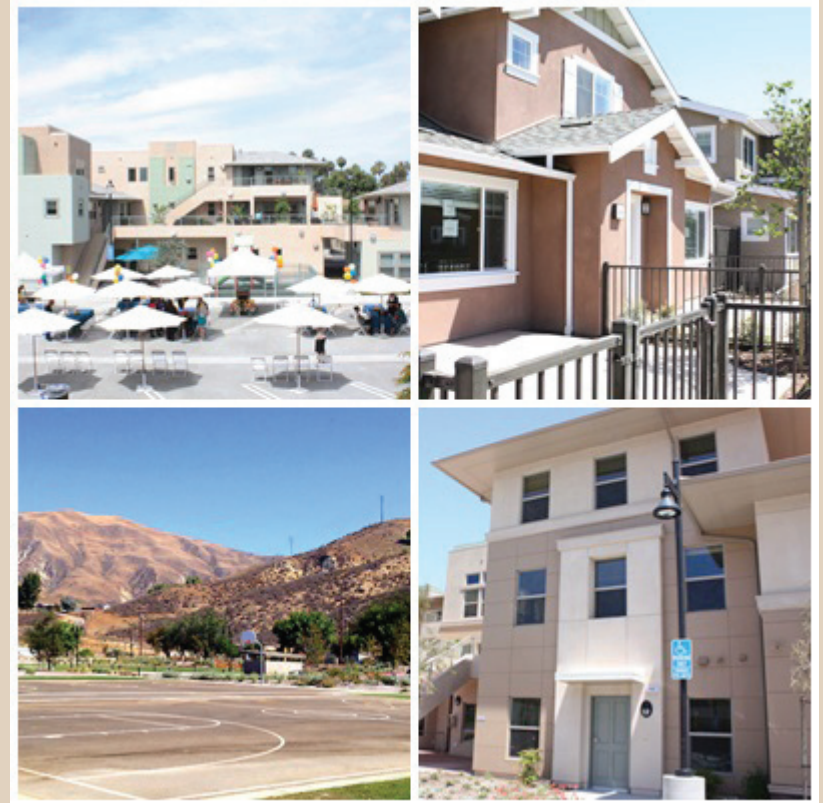
CEDC built four new affordable communities in 2012. Top left: Camino Gonzalez in Oxnard. Top right: Azahar Place in Ventura. Lower left: Valle Naranjal in Piru. Lower right: Paseo de Luz in Onxard.
